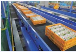
Material handling system delivery and installation project for food distribution center (South Korea)
