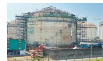
Large-scale refurbishment of a cryogenic tank in Malaysia
