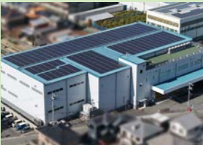
Wakayama Plant Solar Power Installation
