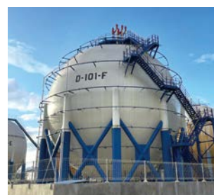
Construction of a spherical tank in Indonesia
