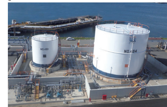
Storage tank for next-generation aviation fuel (SAF)
