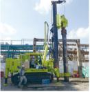
Construction of residential complex Steel pile driving work
