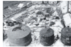
The first ordered tank built at the Showa Sekiyu Muroran refinery
