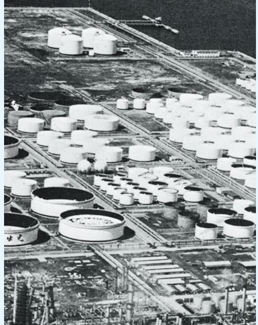
Various types of tanks supplied to the Tokuyama Refinery of Idemitsu Kosan
