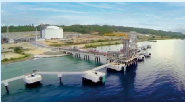
A full-containment tank with a PC (prestressed concrete) outer tank delivered to the Donggi-Senoro LNG project in Indonesia
