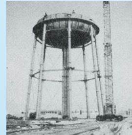
Elevated water tank under construction in Kuwait
