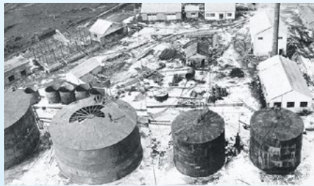
Tank built at the Muroran Refinery of Showa Sekiyu, the first tank order won by the Company
