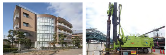
Construction of residential complex
