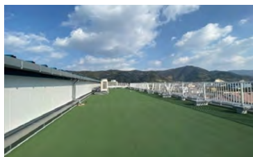
Rooftop of Wakayama Plant No. 3
